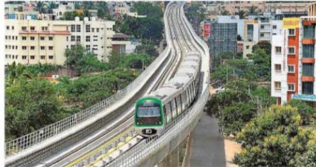
Residents along the line have demanded that BMRCL and BBMP ensure easy access to metro stations. ■ K. MURALI KUMAR
